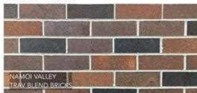
Walls, Soffit (Colonnade)
